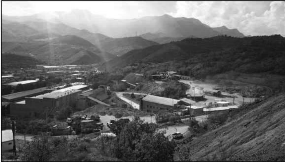
Figure 1: View of the mine site at the Kapan mine and process plant (Polymetal Inc)
